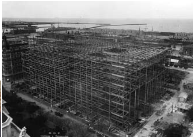
Photographs of the building during the construction showing its metallic structure.
